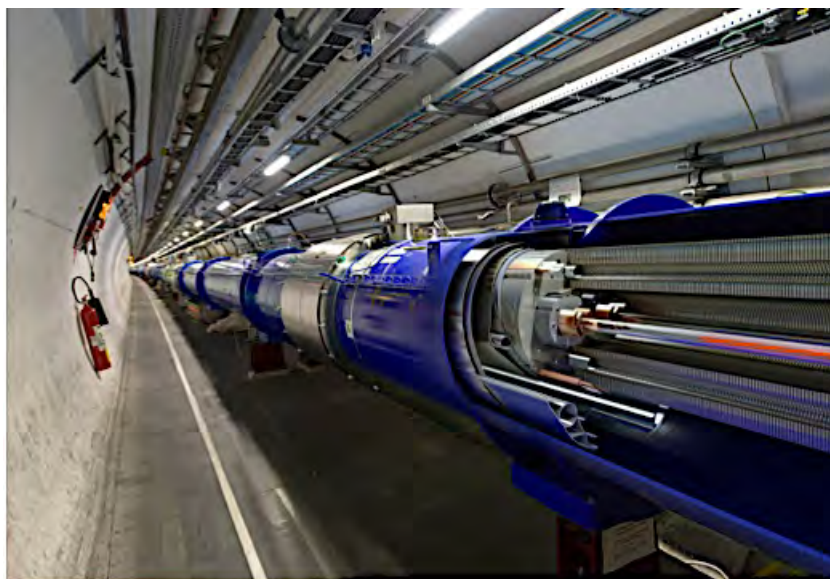
Figure 1- Beam pipe at the LHC 145m under the earth's surface
